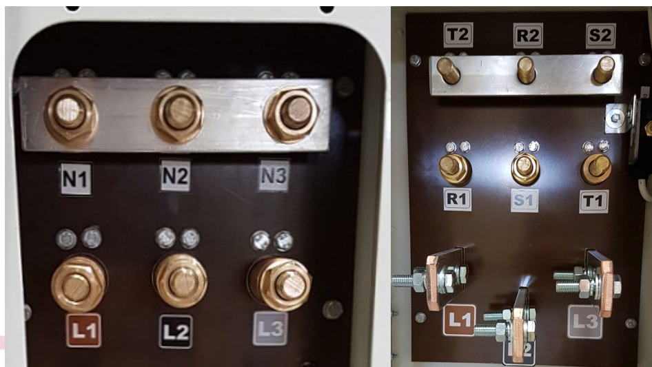
Figure 15- Star/Delta Manual Configuration
